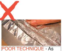
POOR TECHNIQUE - As you can see the spine and tape have air trapped even after hard rubbing.
